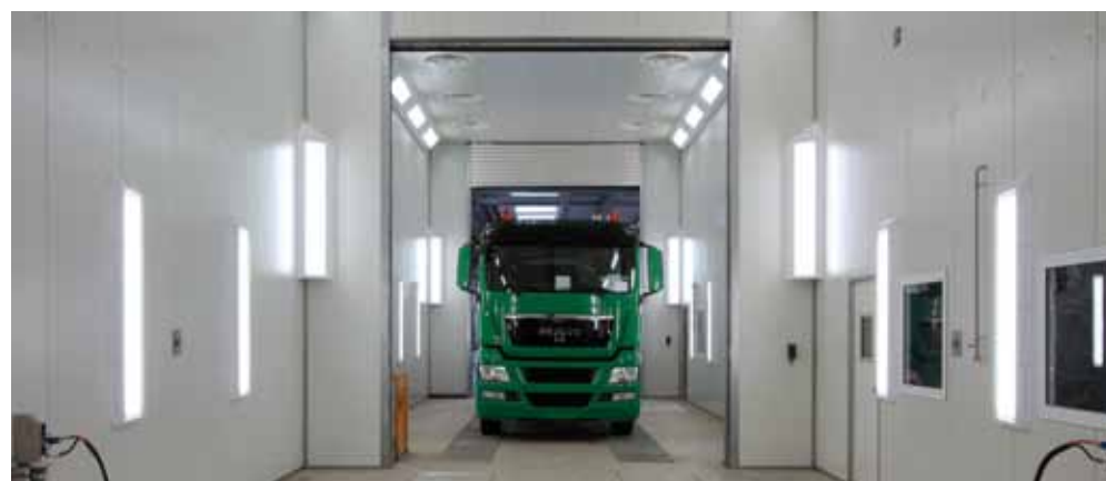
Paint spraying line at company F.X. Meiller in Munich
