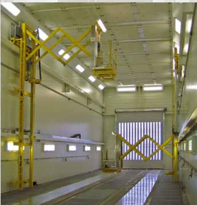
Travelling sidewall-mounted scissor-type lifting platforms in a painting cabin.
