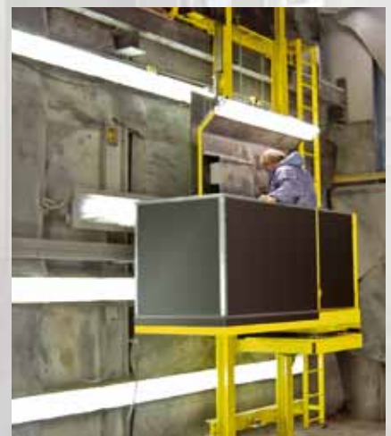
Mobile, swivelling working platform in a blastroom.
