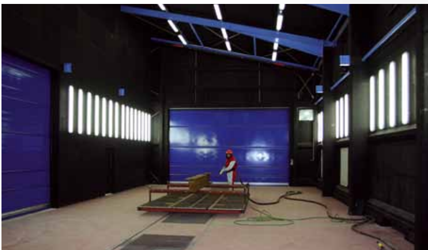
Blastroom for ship components of the Meyer Shipyard incl. partial, pneumatic media recovery.
