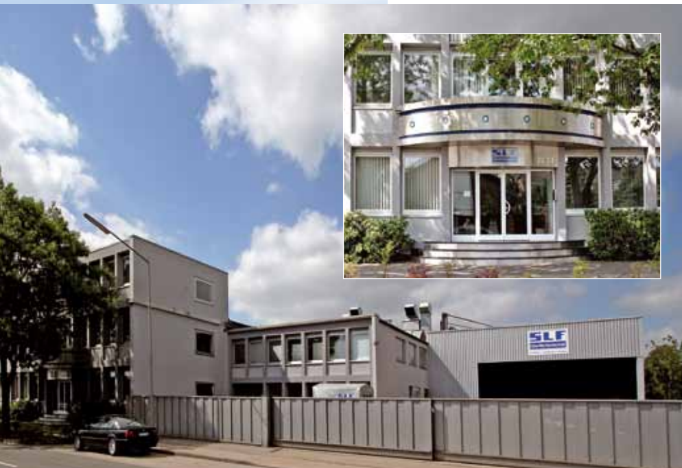
View of SLF Head Office in Greven-Reckenfeld.
