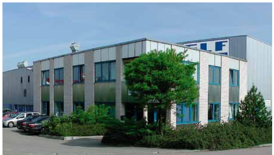
View of factory in Mühlau near Chemnitz (Plant engineering and anti-corrosion center).
