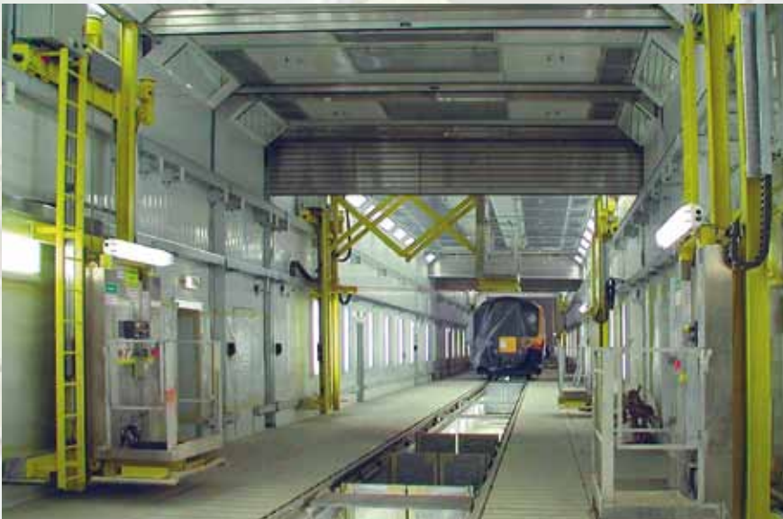
Sidewall lifting platform in a painting cabin for rail cars at Siemens AG Transportation Systems, Krefeld.
