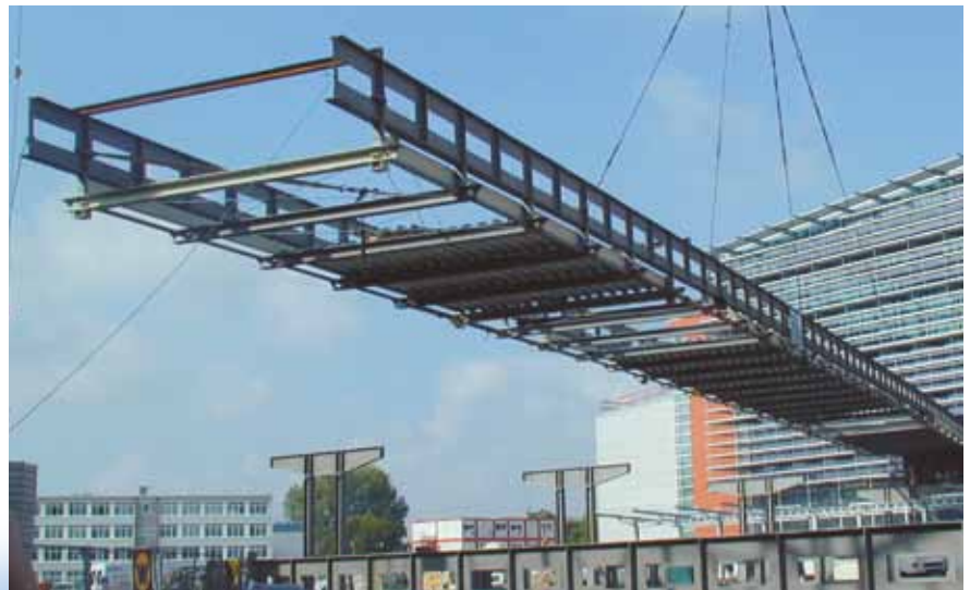
Passenger bridge for the Dresden Airport, processed at the SLF Anti-Corrosion Center in Mühlau.
