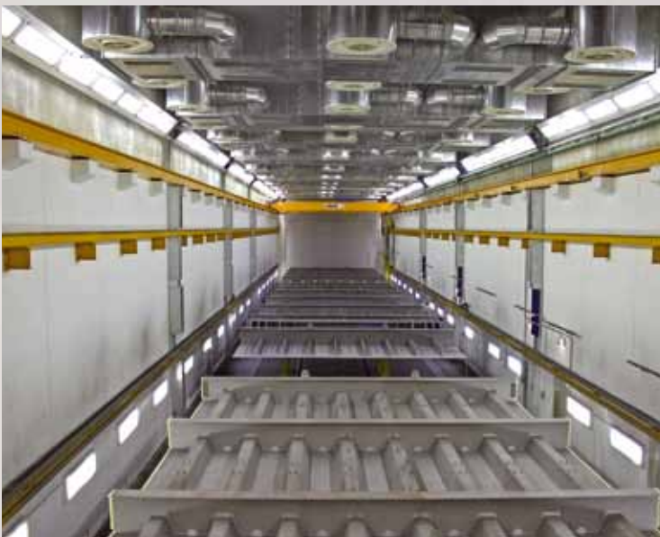
Combined painting and drying cabin with sectional ventilation by means of long-range nozzles for bridge elements.
