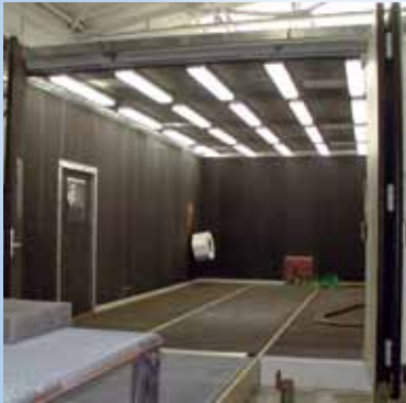
Blastroom with pneumatic media recovery without foundations.
