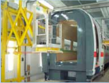
Painting hall with sidewall scissors-type lifting platform.
