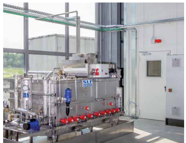
Process water treatment system for a cleaning booth
