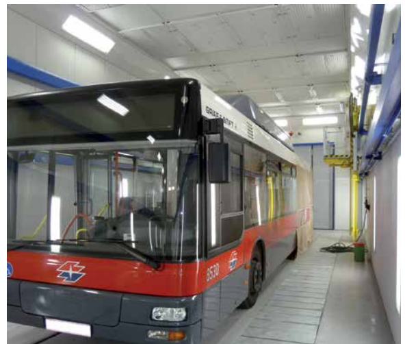
Combined paint spraying and drying booth with lifting platforms
