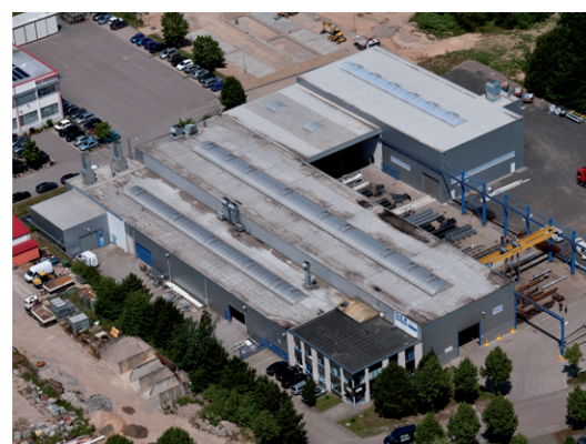
Today's corrosion protection centre in SLF's factory in Mühlau
