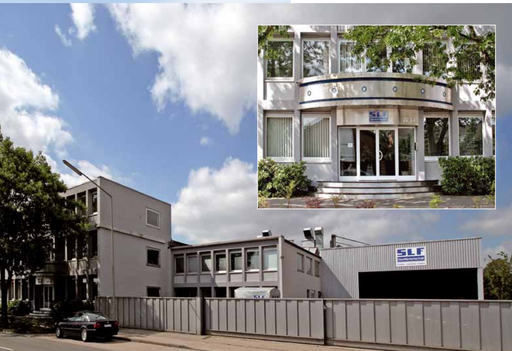
View of SLF Head Office in Greven-Reckenfeld.
