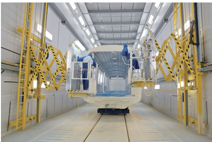
Combined paint spraying and drying booth for rail vehicles with sidewall-guided scissor-lifting work platforms
