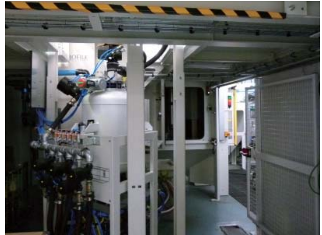
In total each shot peening machine including the filter unit and the compressor unit covers a surface of approximately 70 m 2 . The whole system is encased by sound insulated panels.
